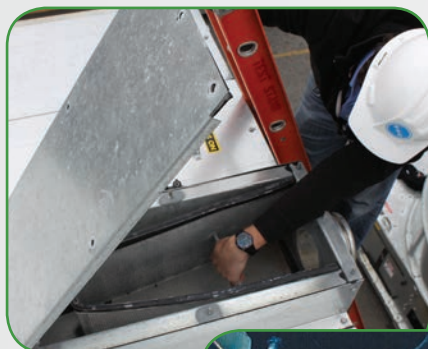
Inlet strainer inspection for Series 1500
